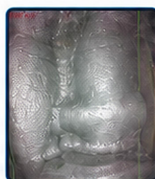
HD inspection imaging
